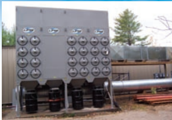
UAS custom designed an extended dirty air plenum to collect particles in all shapes and sizes.
